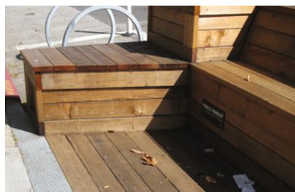
A steel transition plate ensures a flush transition from the curb to the wooden parklet surface.
